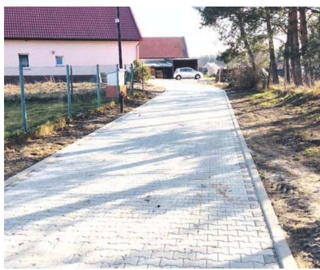
Nowa droga w Starym Górniku
