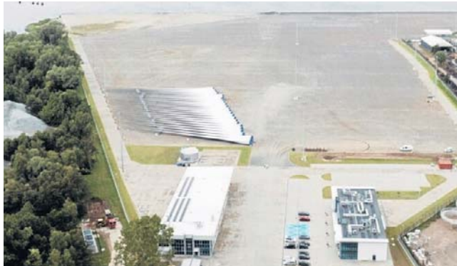
FOT. TERMINAL OFFSHORE WIND
