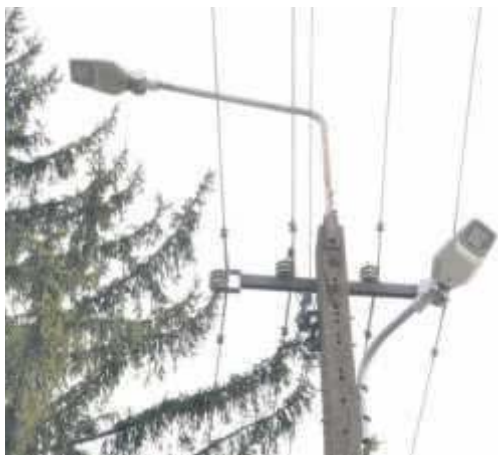
fot. arch. UG Repki
