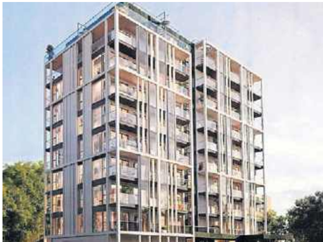
FOT. QUADRA DEVELOPMENT
