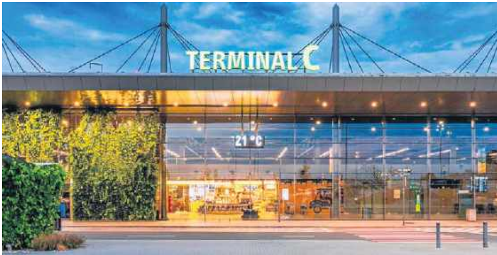
FOT. KATOWICE AIRPORT
