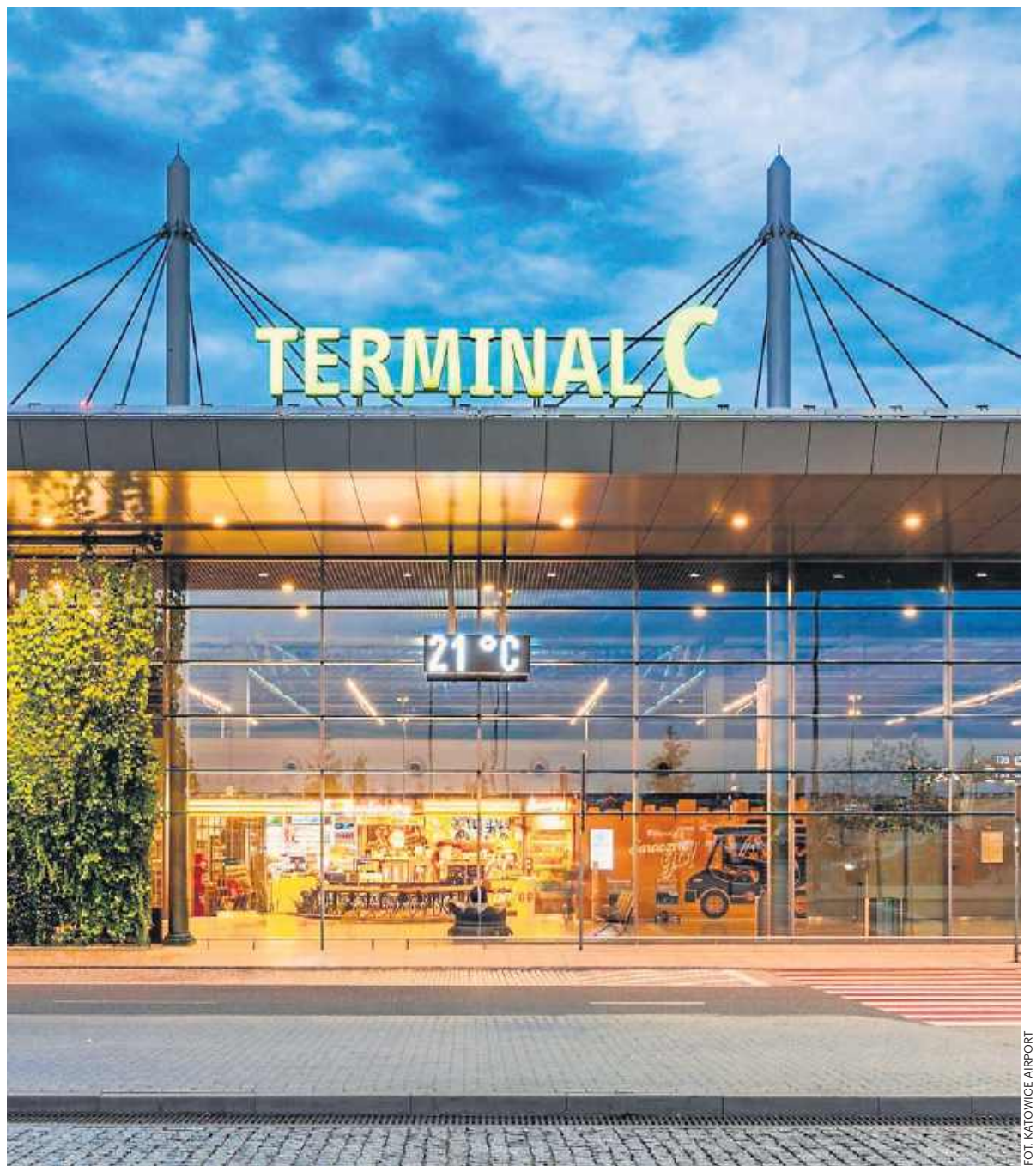
FOT. KATOWICE AIRPORT
