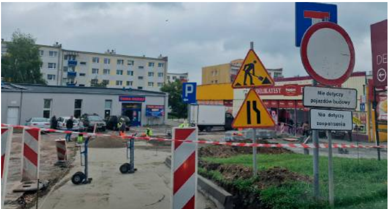
Remont parkingu trwa
